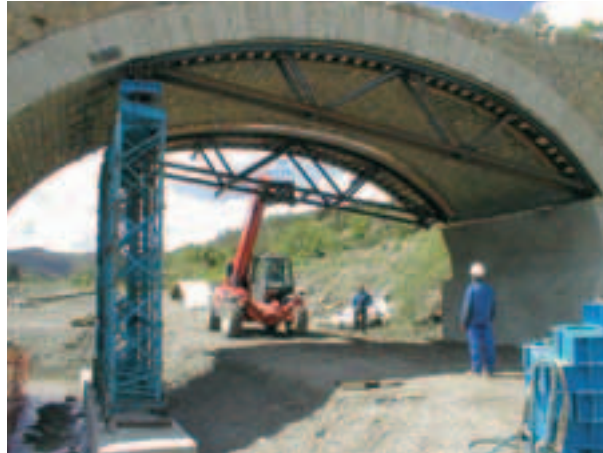
Photo 5 Pose des cintres sous V1 Placing of centres under V1
