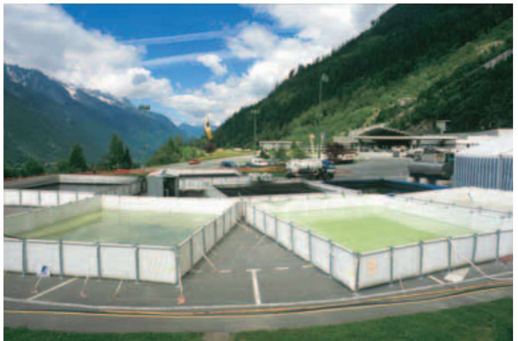
Photo 1 Un chantier de grande envergure A project of impressive scope
