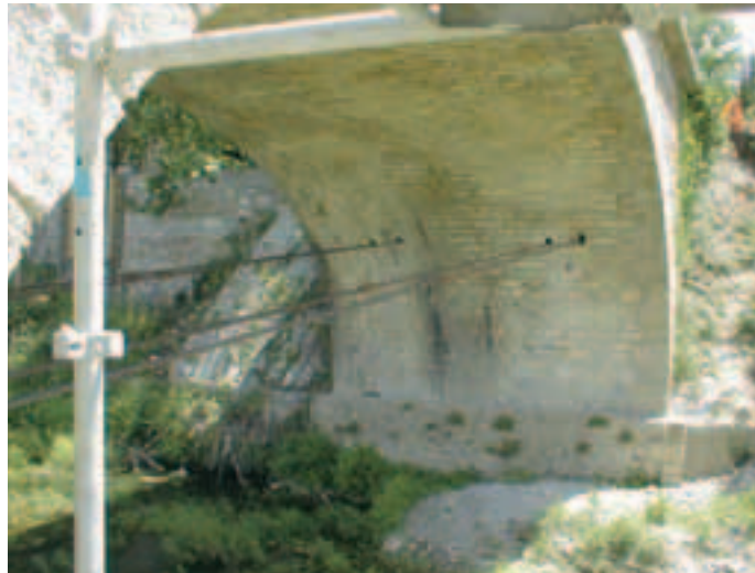
Photo 6 Tirants provisoires voûte V3 Temporary tie-rods for arch V3
