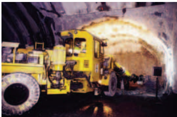
Photo 6 Le forage des abris Drilling for shelters
