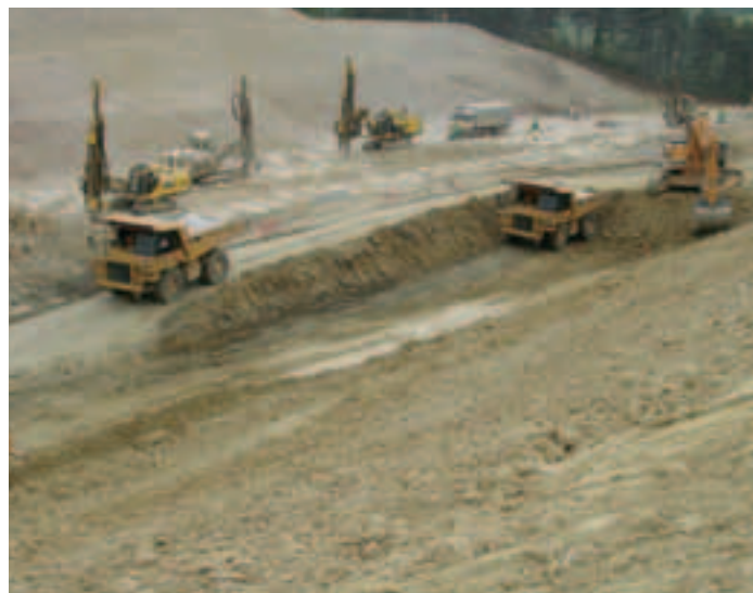
Photo 3 Ateliers de minage - Atelier de terrassement Blasting equipment - Earthworking equipment
