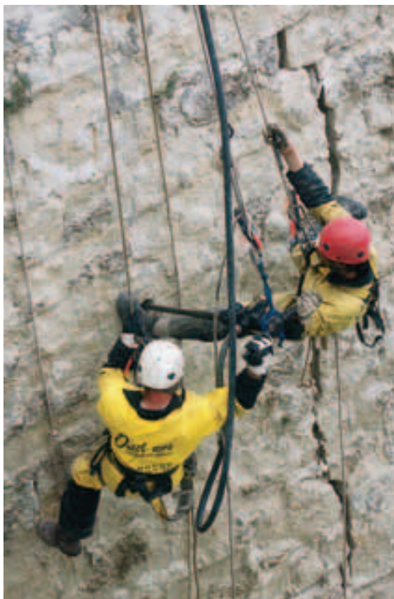
Clouage provisoire Temporary nailing
