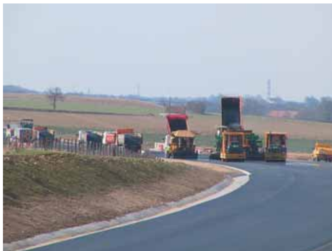
Vue des ateliers d'application du BBTM View of plant for application of very thin asphalt
